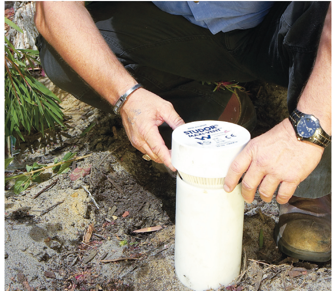
Photo 2: Typical AAV for downstream venting applications
