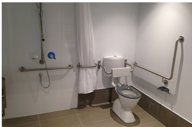
Photo 1: Typical accessible bathroom facilities
