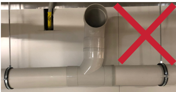
Photo 3: 88° junction on back are not permitted
