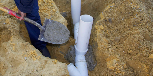
Photo 2: Typical raised inspection opening using square junction
