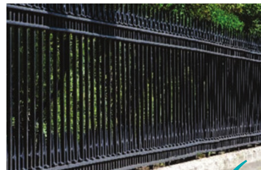
Rail fences provide barriers without compromising surveillance; avoid designs that form ladders. ✓
