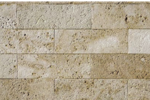
Apply anti-graffiti coatings on porous materials.
