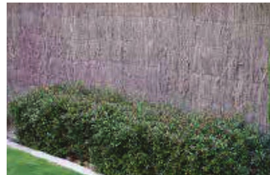
Place hedges, fibrous walls, or dense, thorny vegetation in front of targets to deter vandals.
