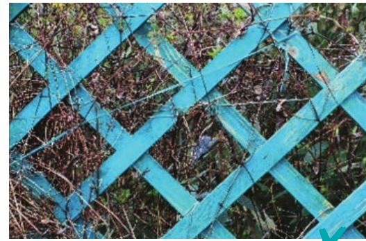
Lattice supporting vegetation can serve as a ladder for offenders. ✗
