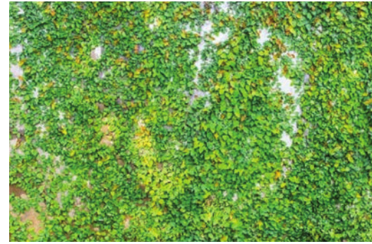
Use creeping vegetation to cover graffiti-prone walls.
