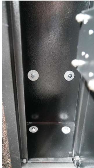
Show all anchor points. A minimum of two anchorage bolts into two separate immovable surfaces ie floor and wall is required
